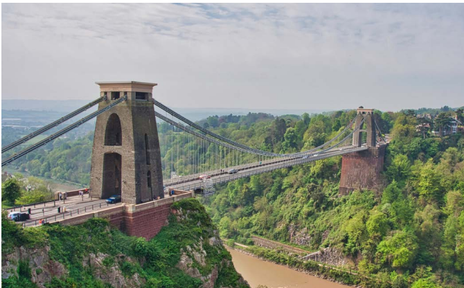
Clifton Suspension Bridge, Bristol
